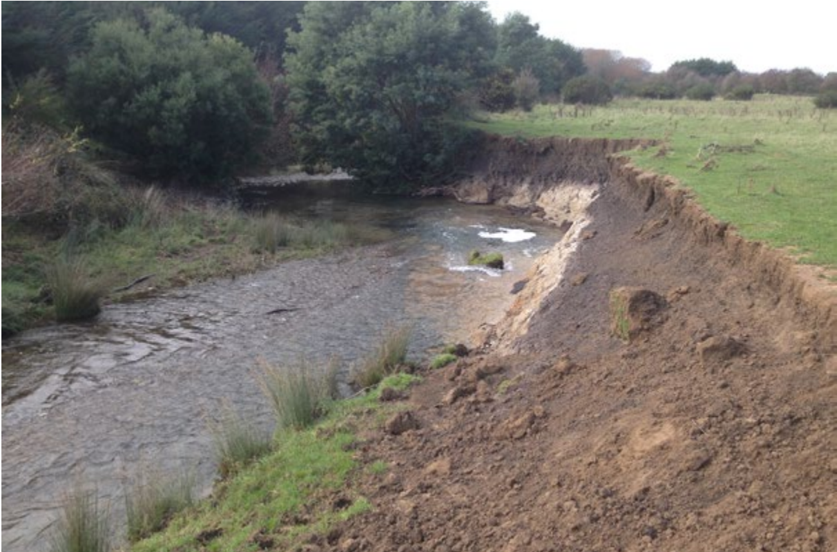
Erosion. Photo: Jesse Webster
