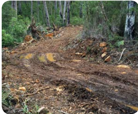
Rutting of roads, particularly in winter, may create potholes that can harbour freshwater diseases. Photo courtesy of Forestry Tasmania.
