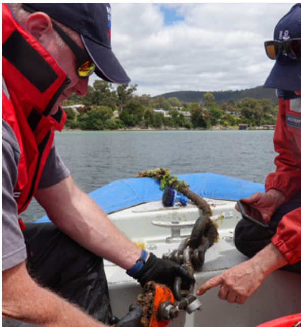
Carrying out maintenance on Environmentally Friendly Moorings.
